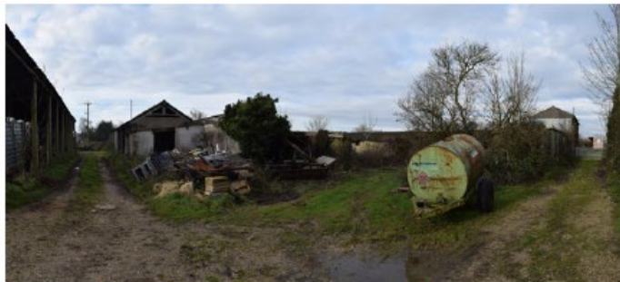
Disused agricultural buildings and equipment in the south of the site.
