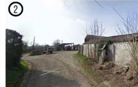
View of the disused agricultural buildings from the access road to Burgate Farm, to the south of the site off of Salisbury Road.
