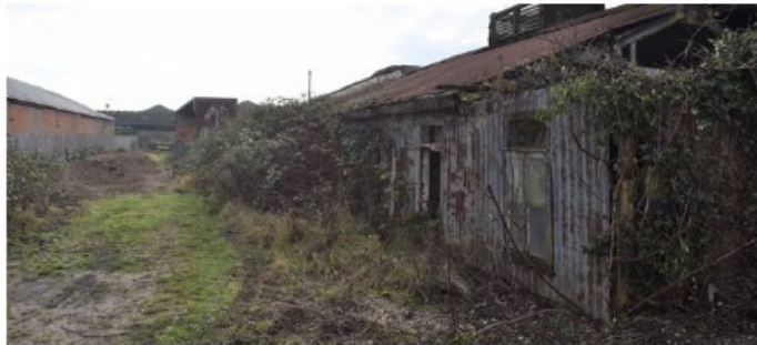
Disused agricultural buildings, with The Fairgate Centre visible on the left.
